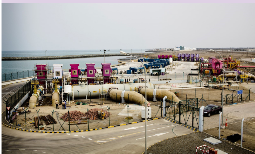
Water management services at Port of Sohar (Oman).
